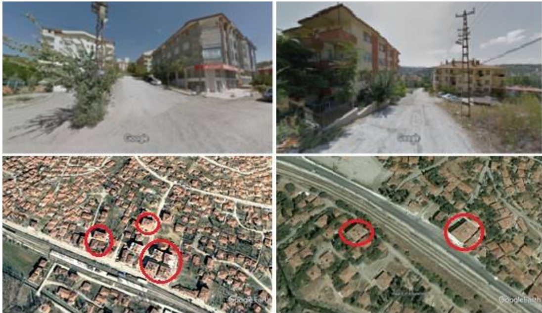
Figure 62. Apartment Blocks and Urban Fabric in Project Area
