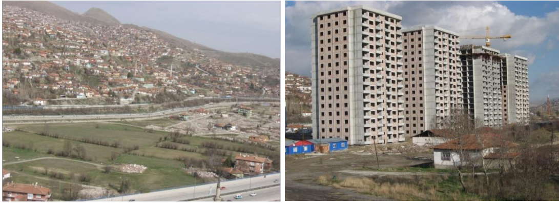
Figure 67. Views of Construction Site in Üreğil (from 2007 to 2010)
